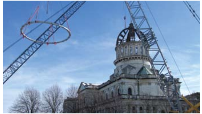
The dome being dismantled piece by piece
