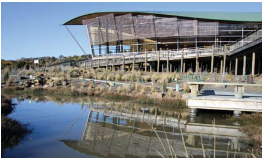
Glazed over – the award-winning windows of Orokonui Ecosanctuary Visitor Centre.
